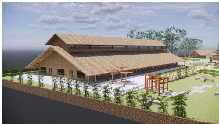
Figure 62 Double roof System
