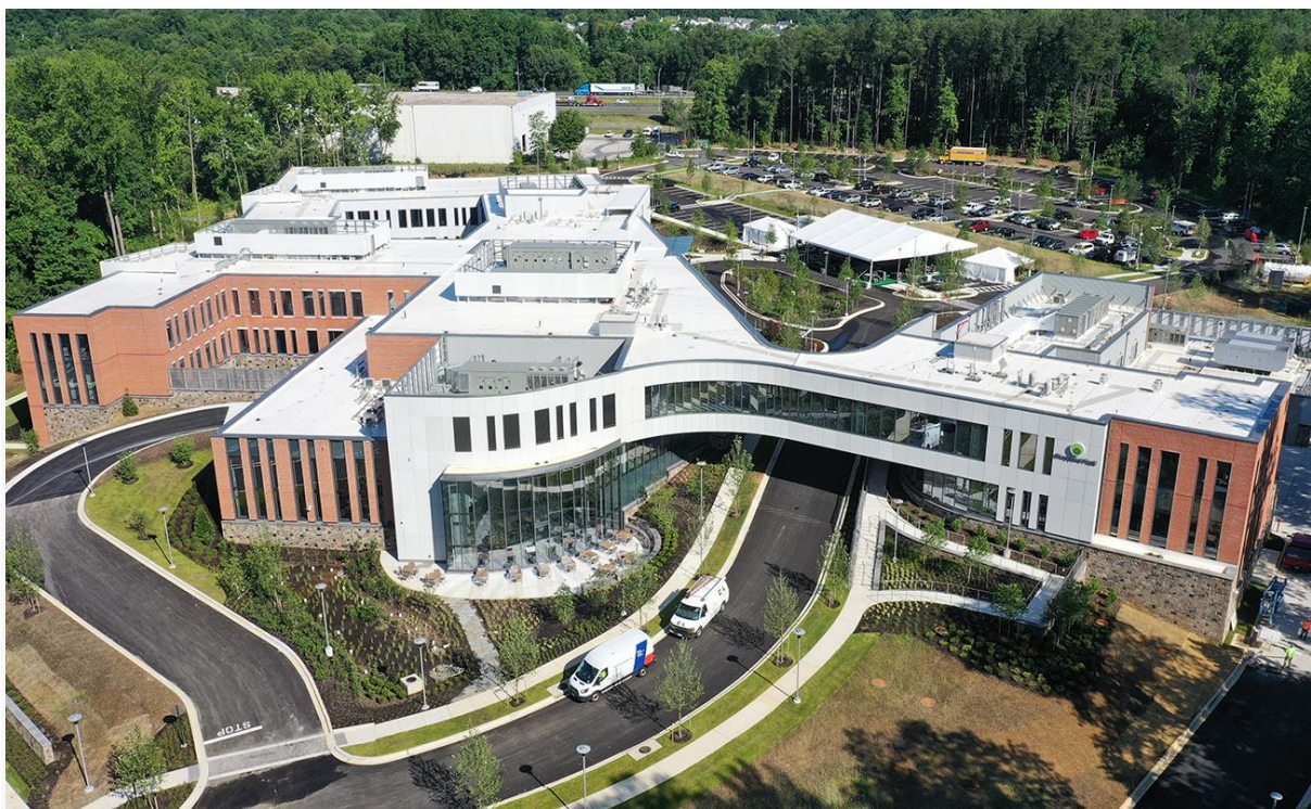
Figure 30 Renovation of the Institution / Source: Lewis Contractors
