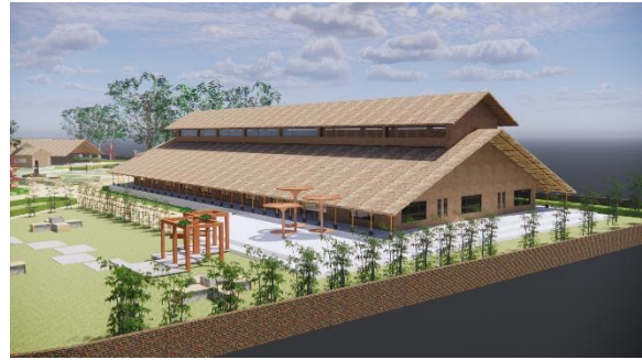
Figure 59 Overhangs and Colonnades and its impact in passive heating/cooling
