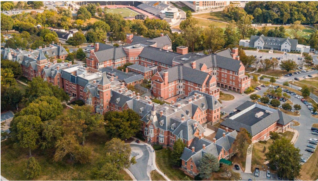
Figure 29 Sheppard Pratt Hospital Baltimore, USA /Source: Sheppardpratt.org
