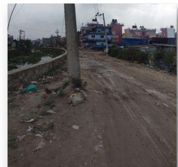
Figure 4-10 8m road at east
