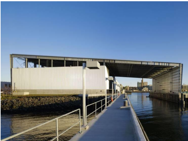
Figure 3. 29 Barges loading and unloading area (Arch daily)
