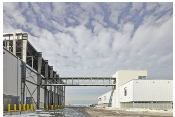
Figure 3. 33 View of bridge that connects education center with processing block (Selldorf Architects)
