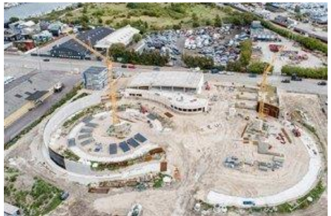
Figure 3. 43 Sydhavns recycling center during construction phase (Strabag)
