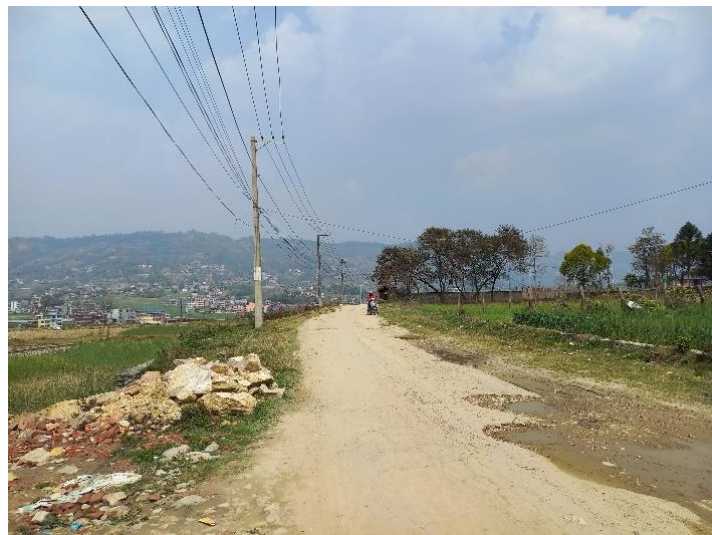
Figure 4. 7 Road condition around site
