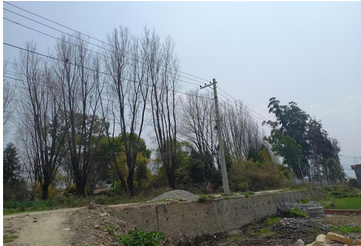
Figure 4. 6 Electrical lines running parallel to the site
