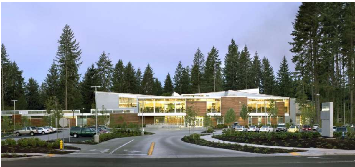
Figure 3.1.2. Entrance Image of Firstenberg Community Center
