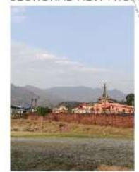
EXISTING BOUNDARY WALL (EAST VIEW)
