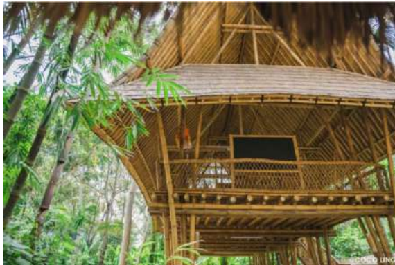
Figure 2. 60 The classic post and beam method in bamboo
