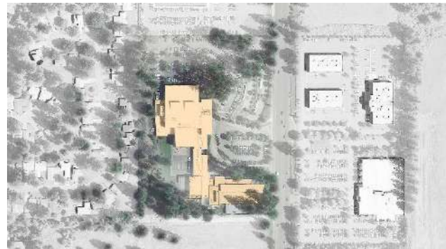
Figure 3.1.1. Top View of Firstenberg Community Center
