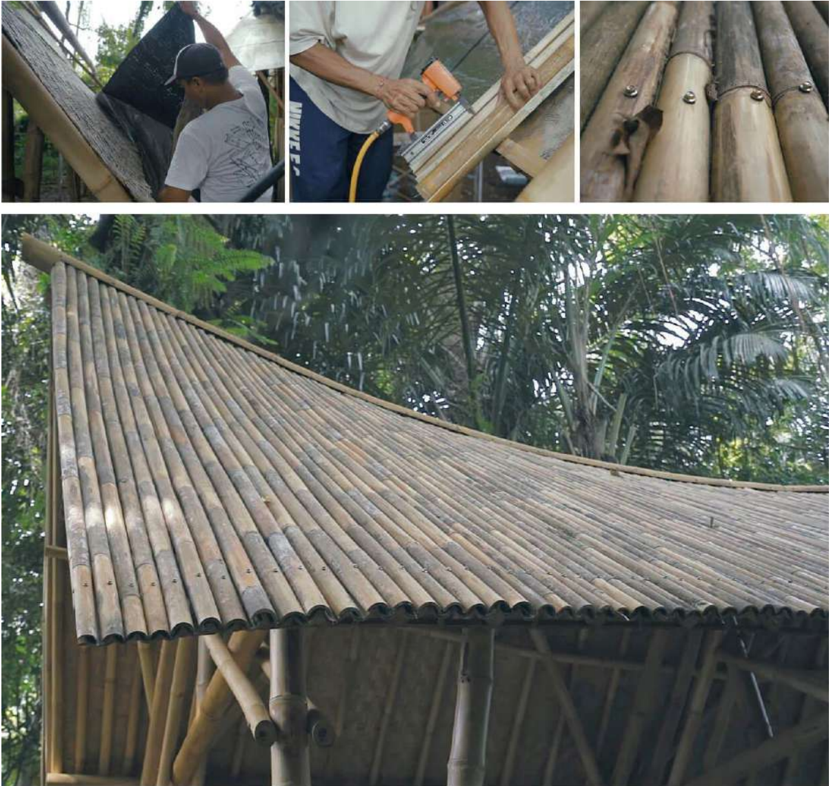
Figure 2. 66 Halved Bamboo roofing
