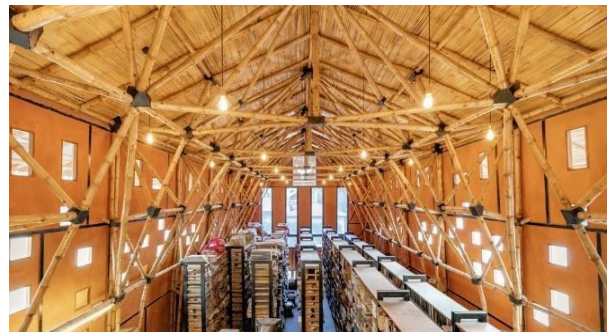
figure 3.1 x Bamboo roof structure
