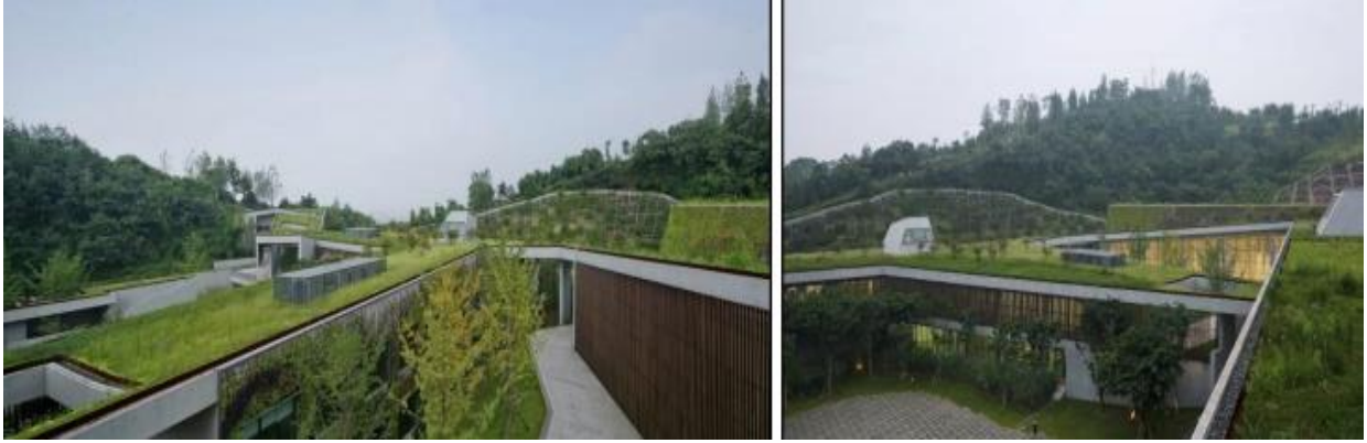
Figure 3.2 u The Undulating Green Roofs of Building
