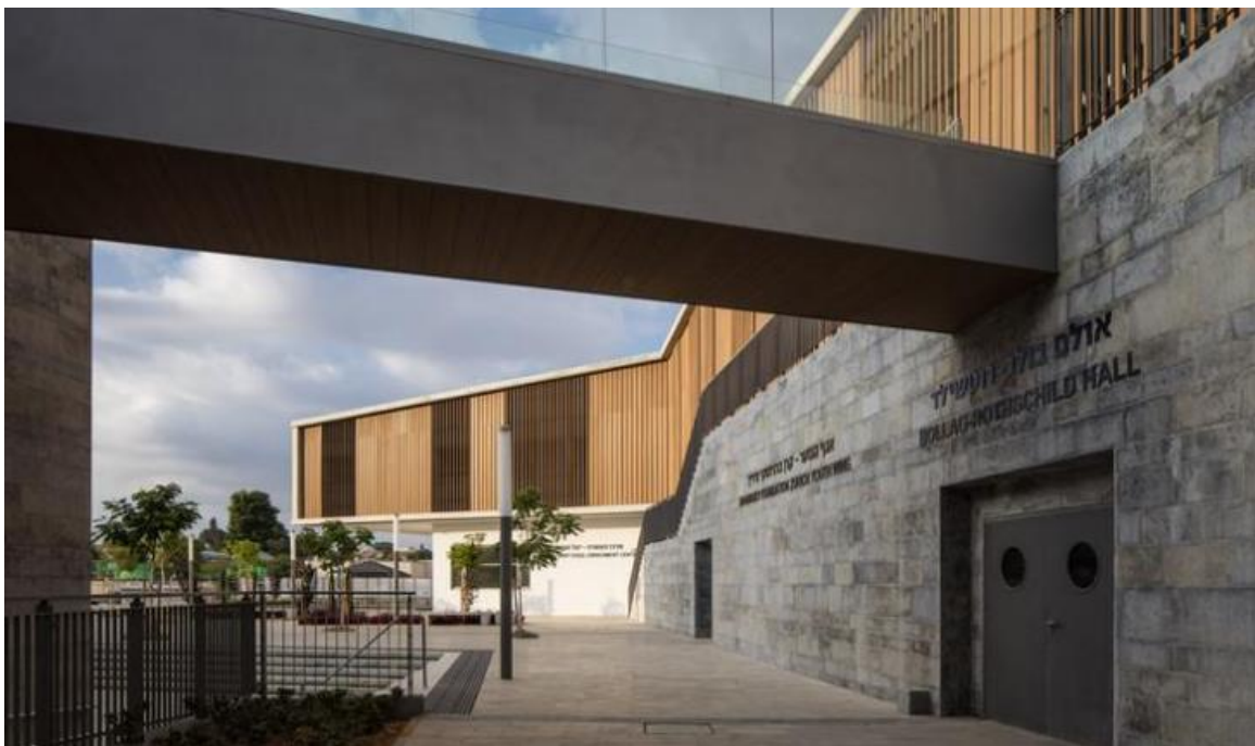
Figure 3.2 j Main building of center
