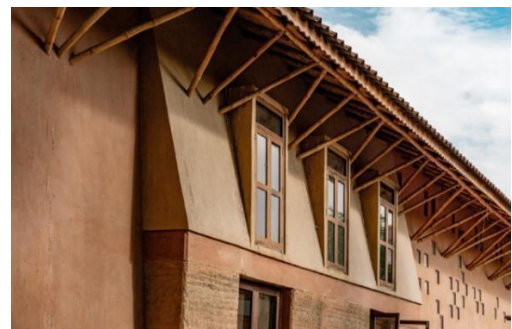
figure 3.1 bb Windows and exterior of library
