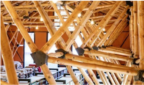
figure 3.1 aa Bamboo joints
