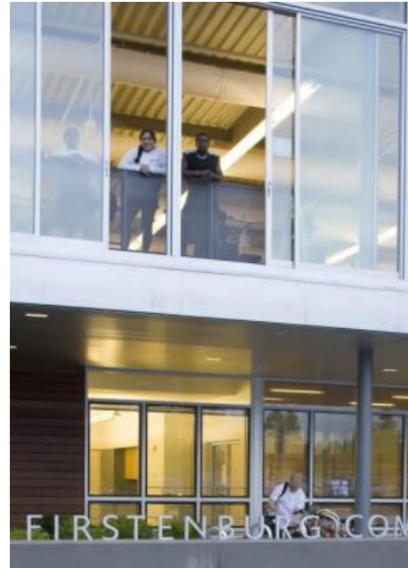
Figure 3.2 h Large openings in wall
