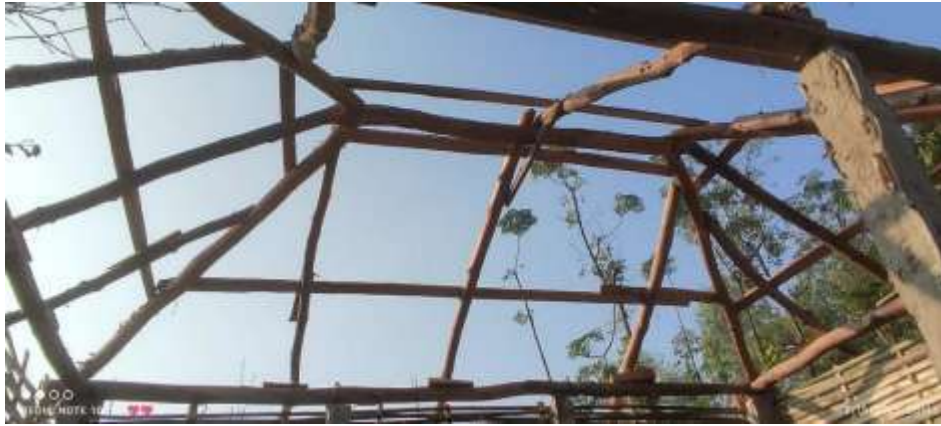
Figure 7- Roof in Tharu house
