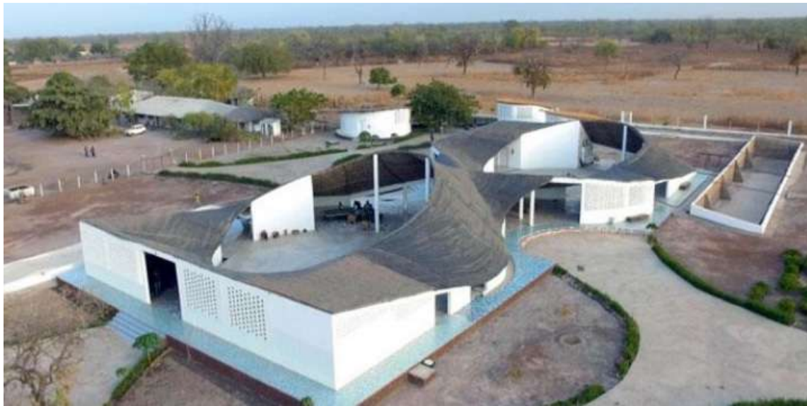
Figure 82- Aerial View of Cultural Centre, sinthian, Senegal
