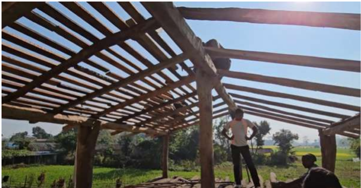
Figure 6- Roof of building
