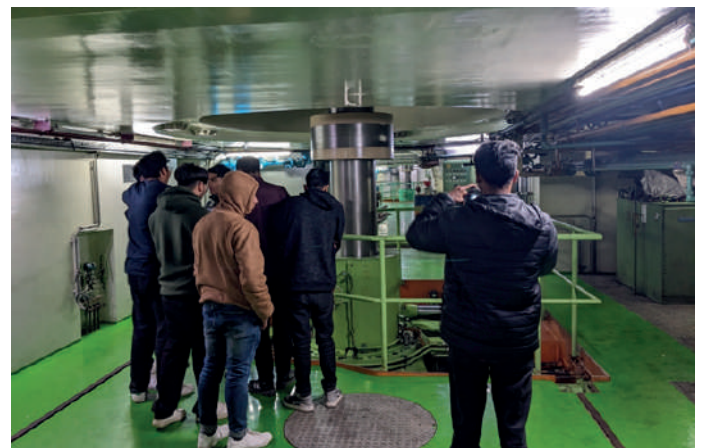
At Lower-Marsyangdi Hydropower
