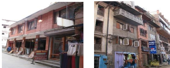
Fig. 9. Brick masonry with cement mortar (BC)
