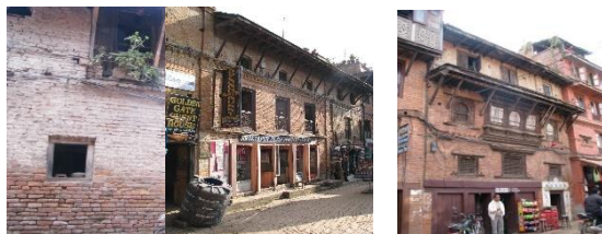
Fig. 10. Brick masonry buildings with mud joints (BM)
