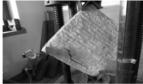
Fig. 12 Propagation of cracks
