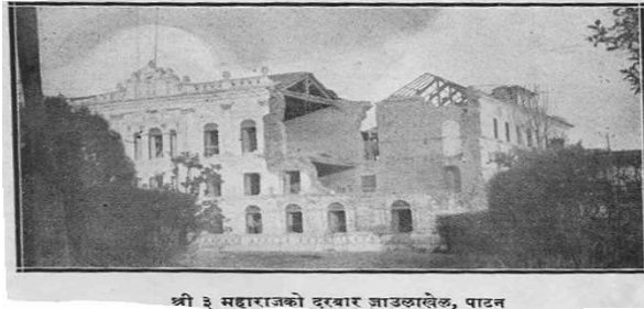
Fig 14. Jaulakhel Darvar after 1990 BS earthquake.
