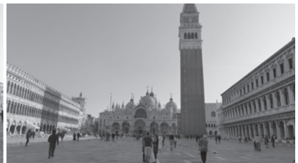
St Mark's Campanile
